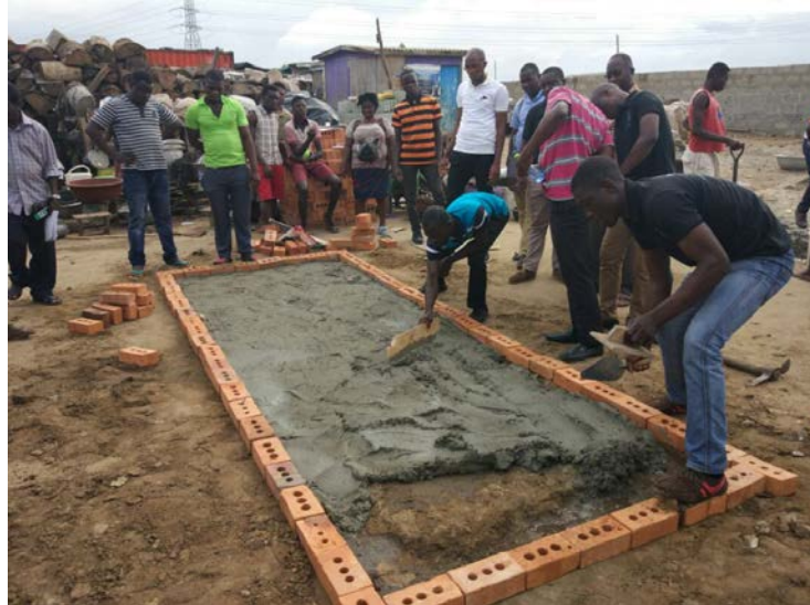
Figure 11: Participants of the technical training constructing samples of the Ahotor oven to the new specifications
