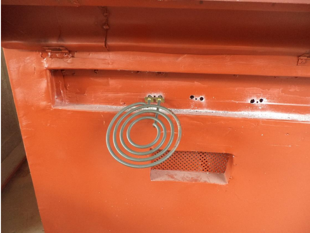
Figure 28: Installation of heating coils
