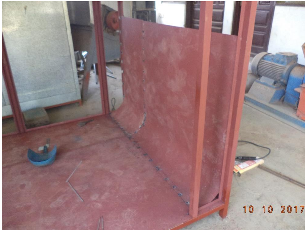
Figure 17: Installation of right Inner plate
