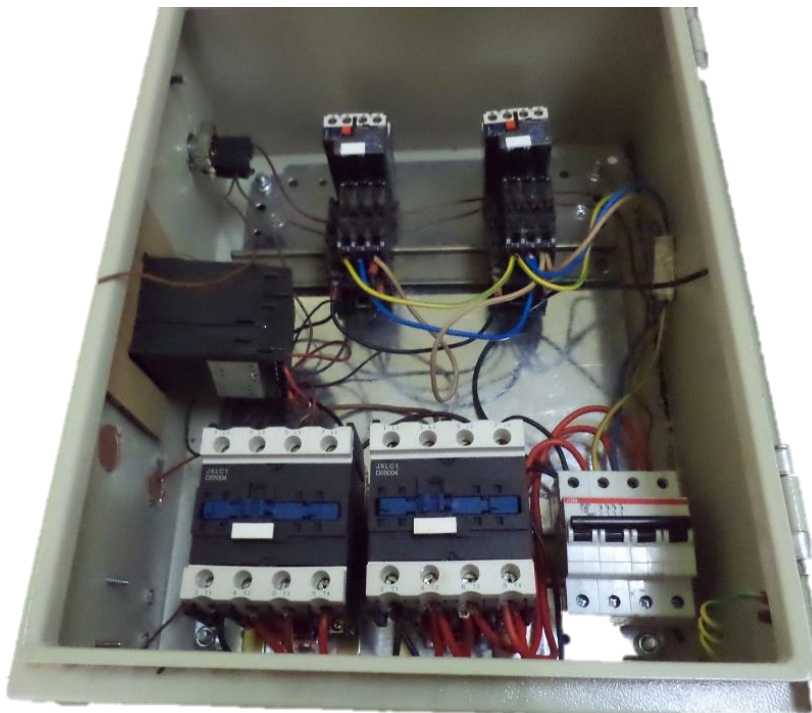
Figure 23: Wiring of control board
