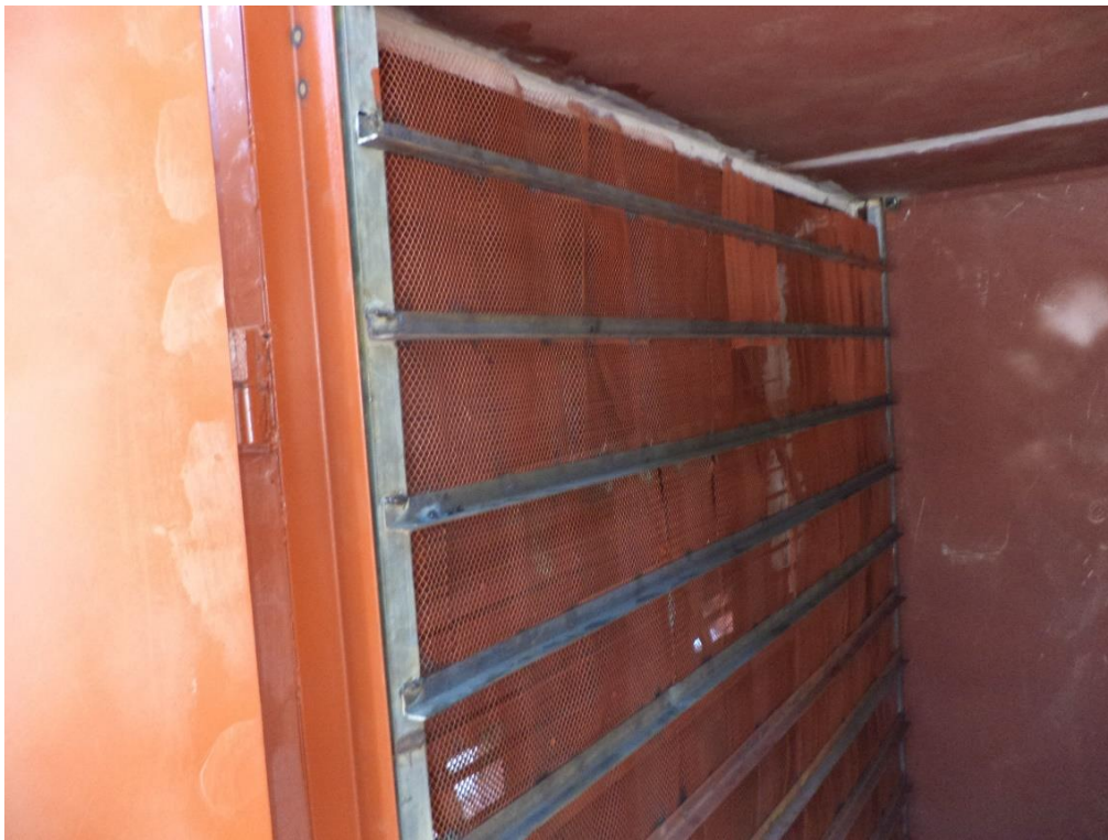
Figure 29: Installation of tray holders inside Dryer
