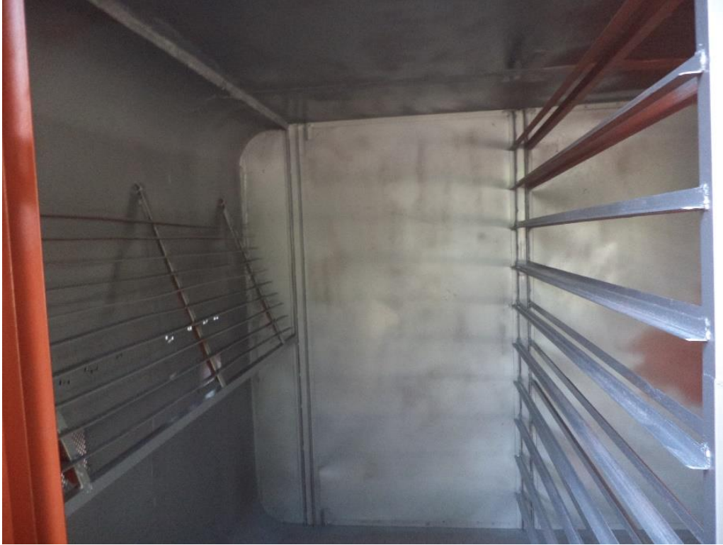
Figure 30: Installation of coil guards and spraying of inner Dryer chamber
