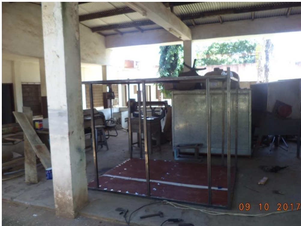
Figure 11: Construction of dryer base
