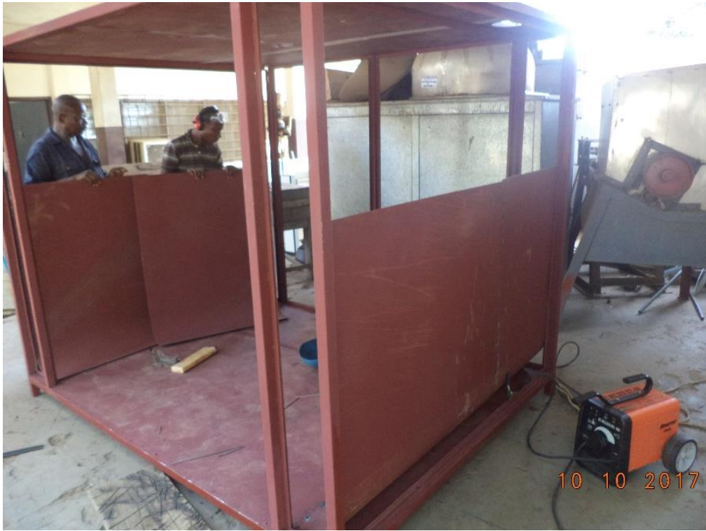
Figure 16: Installation of left inner plates
