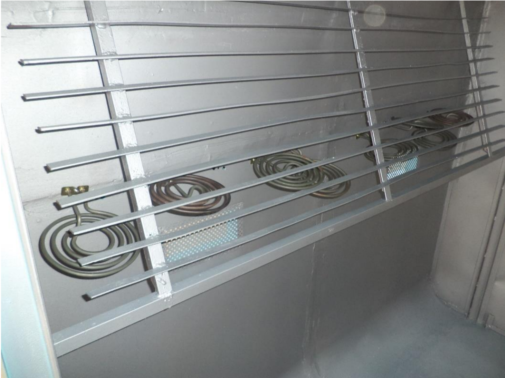
Figure 31: Complete installation of heating coils
