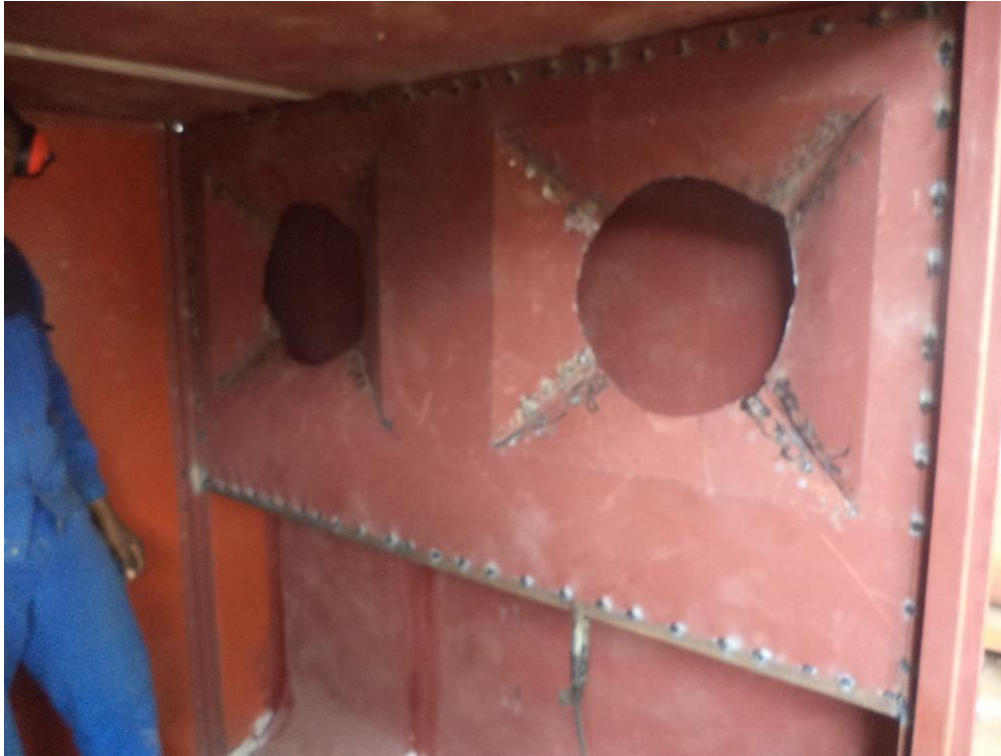
Figure 19: Installation of fan duct threshold
