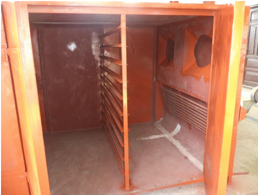
Figure 21: Further application of anti-rust paint to exposed metal parts
