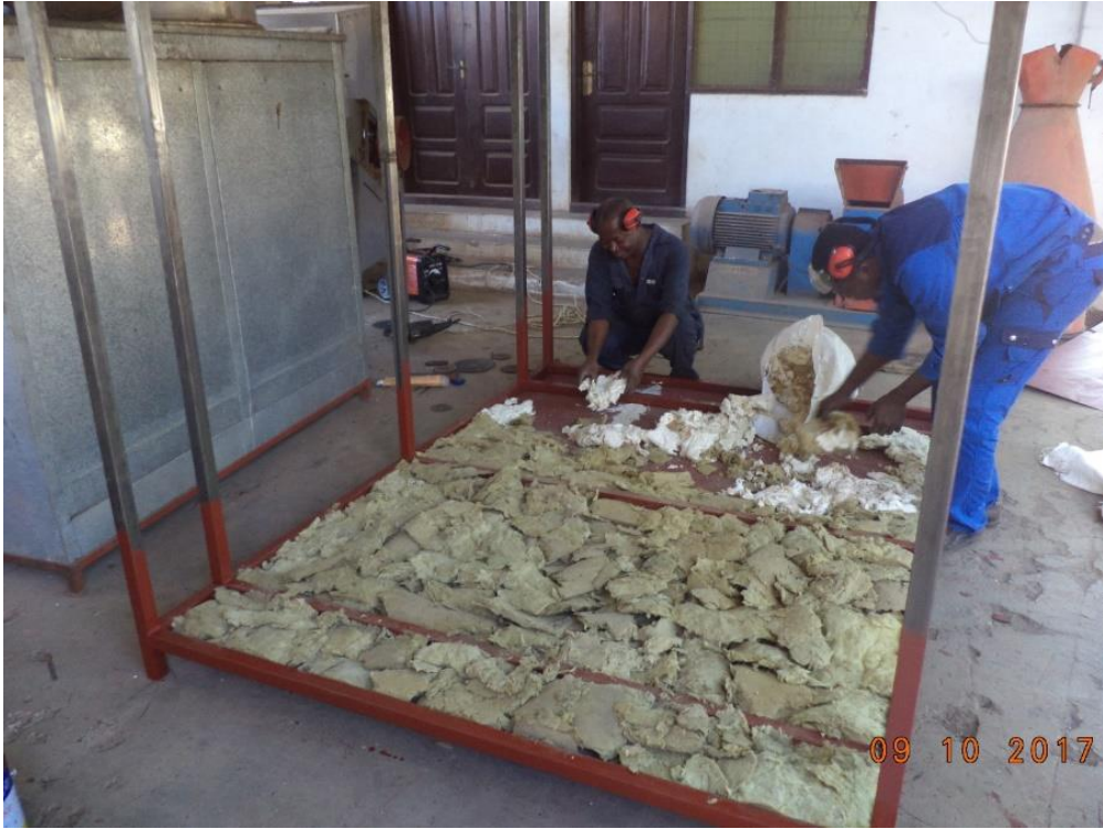
Figure 12: Insulation of dryer base
