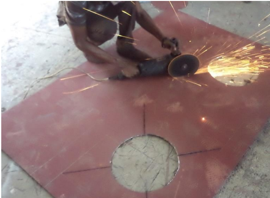
Figure 14: Cutting of Fan duct threshold
