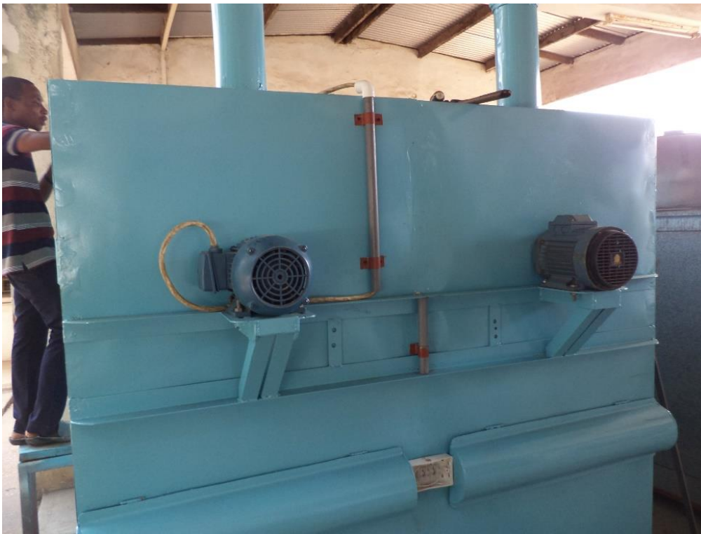
Figure 33: Mounting of Electric Motor
