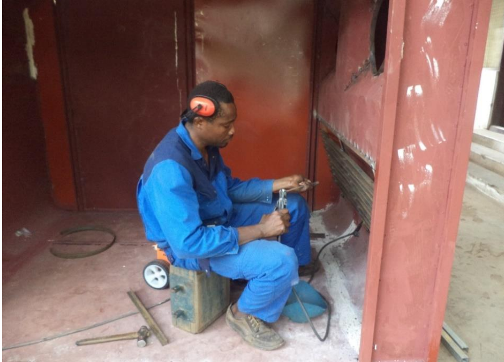
Figure 20: Installation of dryer buffers
