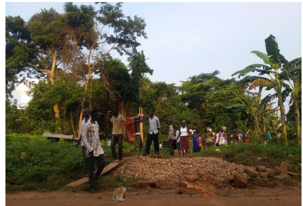
Participants leaving construction site
