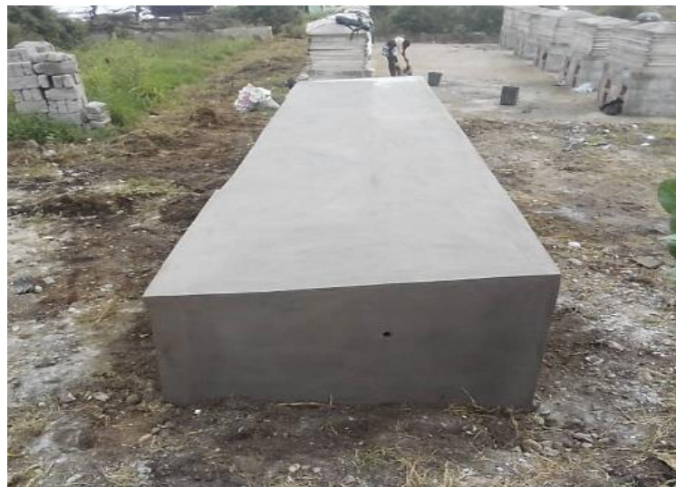
Figure 5 Drying platform depicting gentle angle of slope
