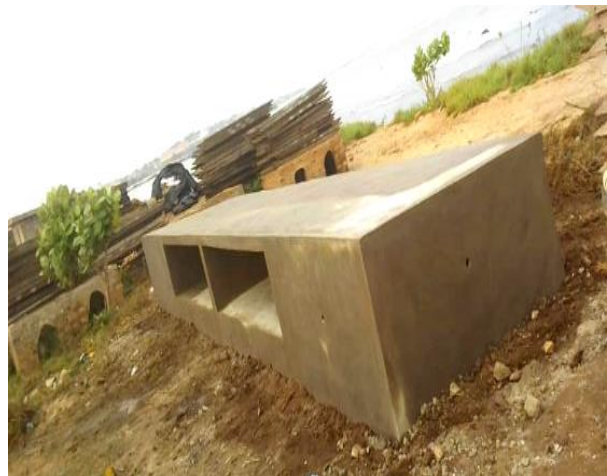
Figure 10 Concrete platform with storage space for racks
