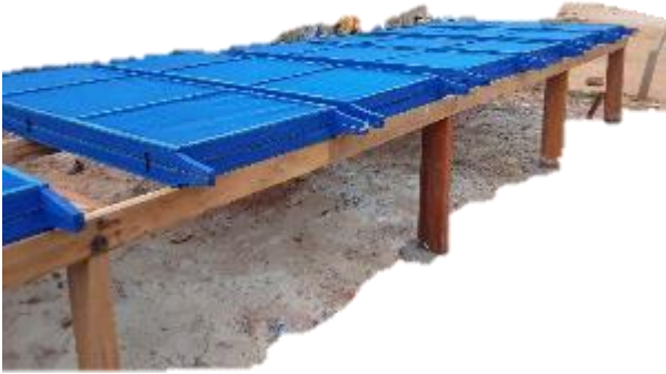
Figure 11a Side view of Timber platform dryer
