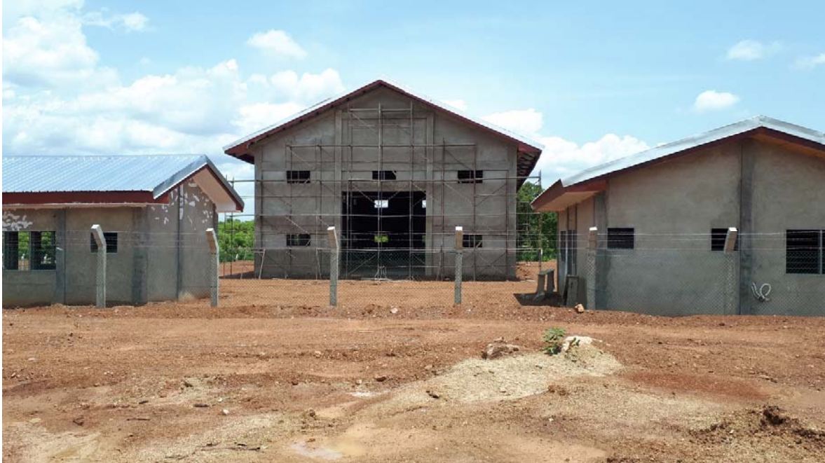
Figure 3-10: Warehouse under construction near Sabuli in Upper West Region, May 2019
