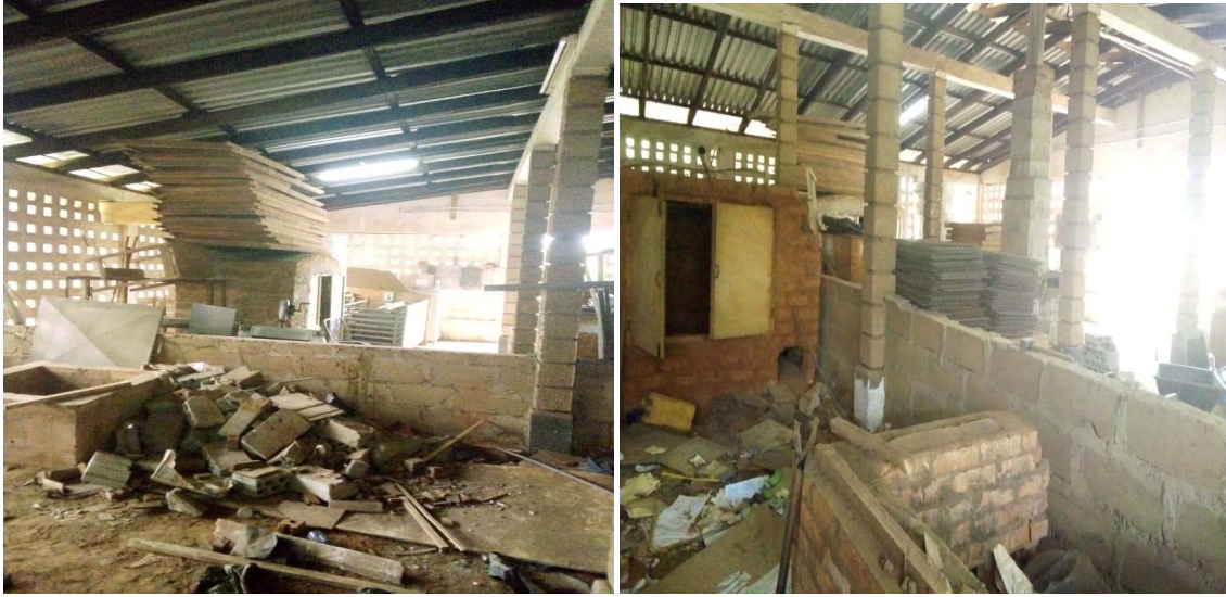
Fig 1 Processing Hall at the start of renovation works.
