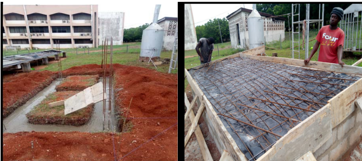
Fig. 1 Construction of drying platform at CSIR-FRI
