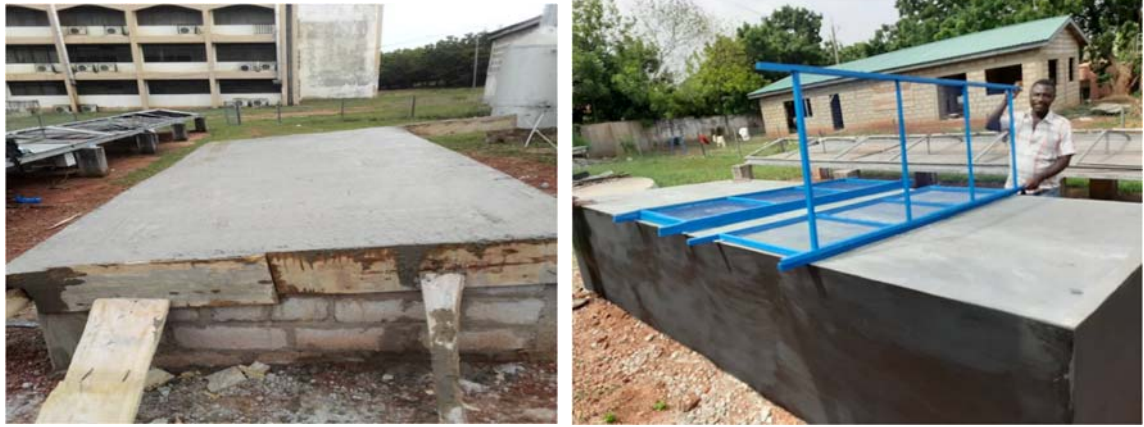
Fig 2. Completed drying platform and rack
