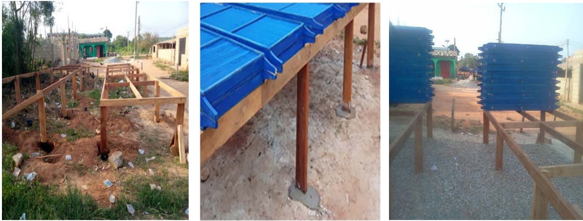
Fig 20. Construction of platform and drying racks at Moree
