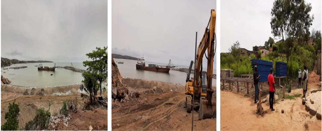
Scenes from the landing beach at Moree and drying platform site
