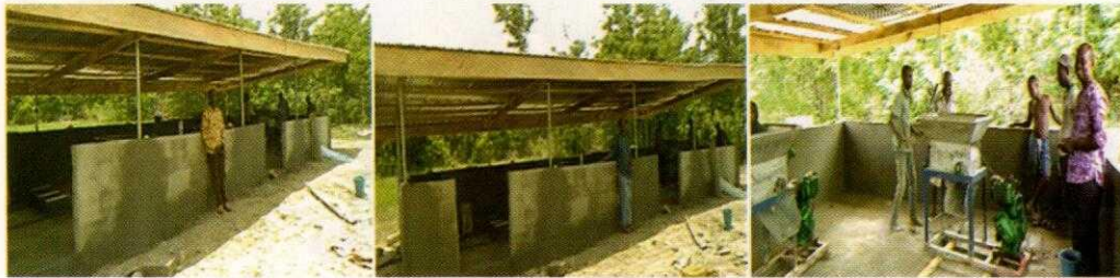
Constructed housing and installation of WAAPP equipment
