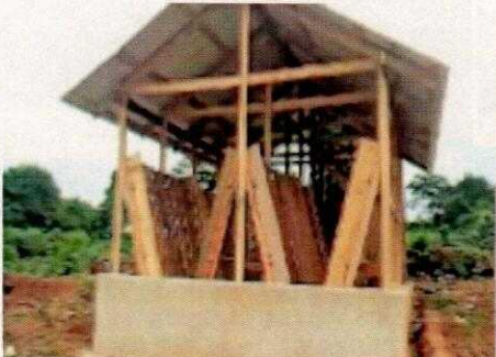
Cropping house Ayumso showing internal arrangements
