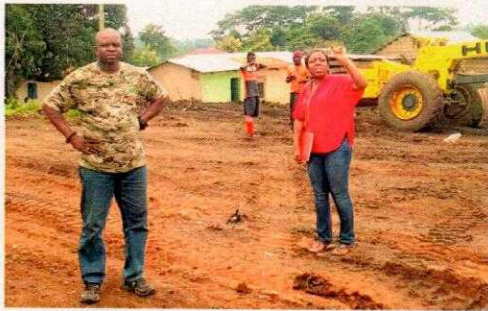
Site grading at Badiako
