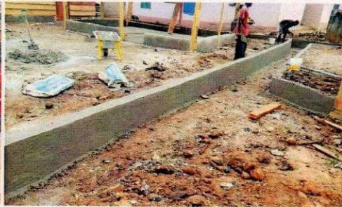
Gutter construction at Badiako
