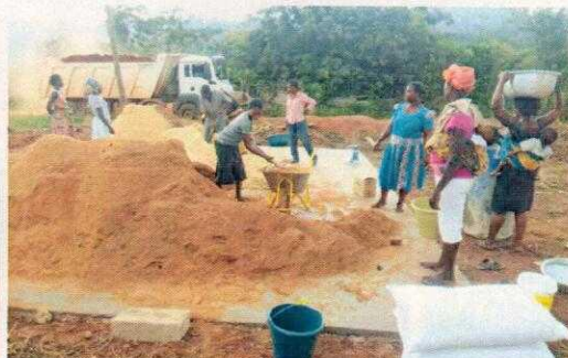
Compost preparation and on composition platform
