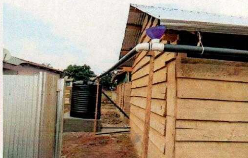
Polytank installed and connected to rain gutters
