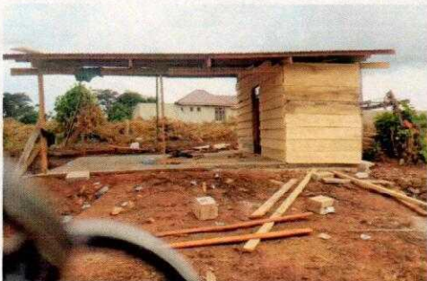
Bagging shed and store constructed at Ayumso
