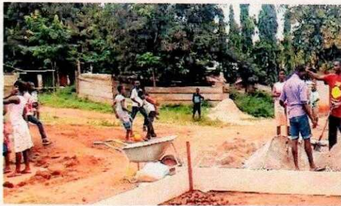
Commenced construction at Badiako
