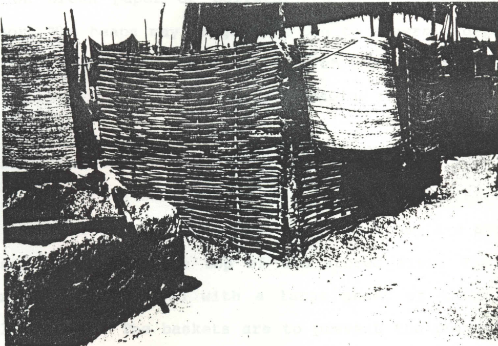
Fig 15. Pictures showing a fenced yard traditional storage structure constructed with woven sticks.
