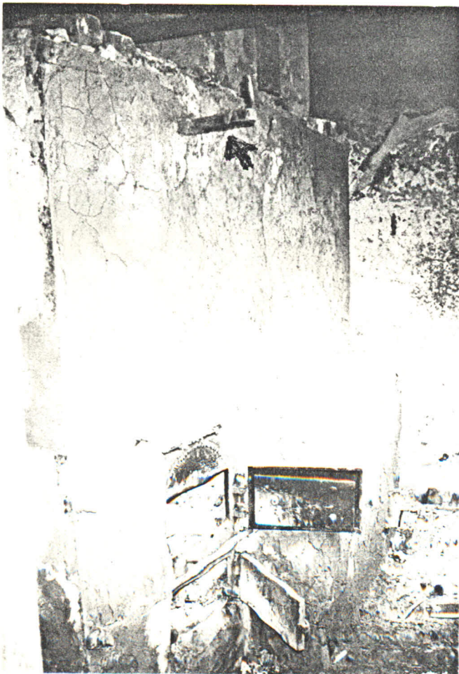
PLATE 7B: The firing chamber of the metal brick oven. It is provided with a chimney.
